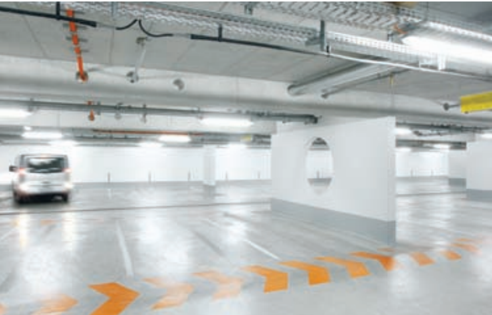
Bavaria underground car park, Munich/Germany
